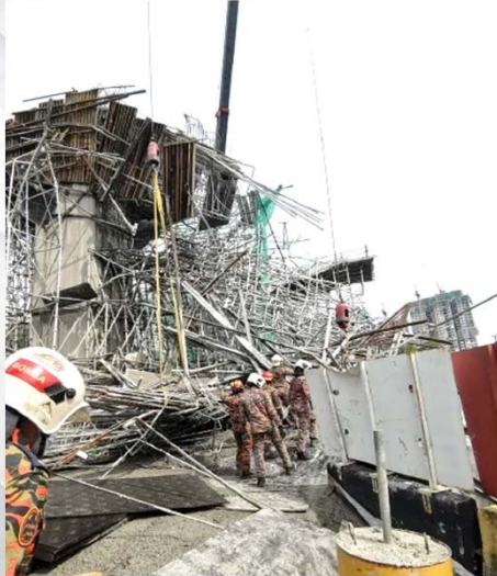
Falseworks Collapse
