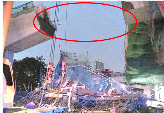
Falseworks Collapse
